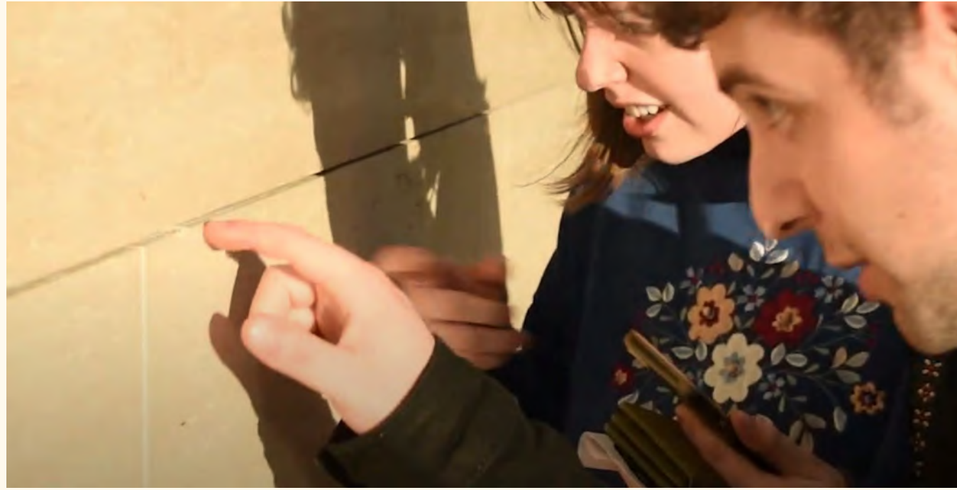
Above/ Image by B. Nishikawa Inspecting a wall at the Ara Pacis Museum, Rome
