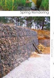
Gabion retaining wall Source: http://milkwood.net/2011/05/06/rock-science-building-ourgabion-wall/
